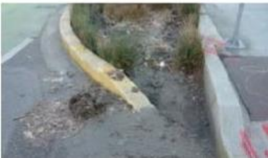
Inlet with basin full of sediment
